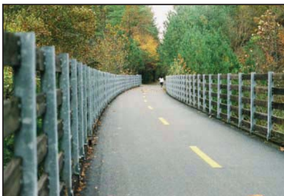
Multi-use bridge in Atlanta
