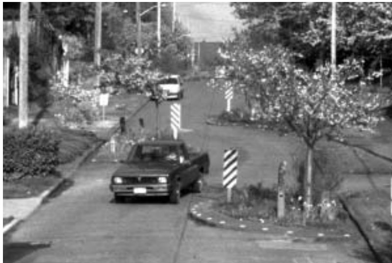
The chicanes pictured above narrow this residential street to one lane and require traffic to move slowly.
