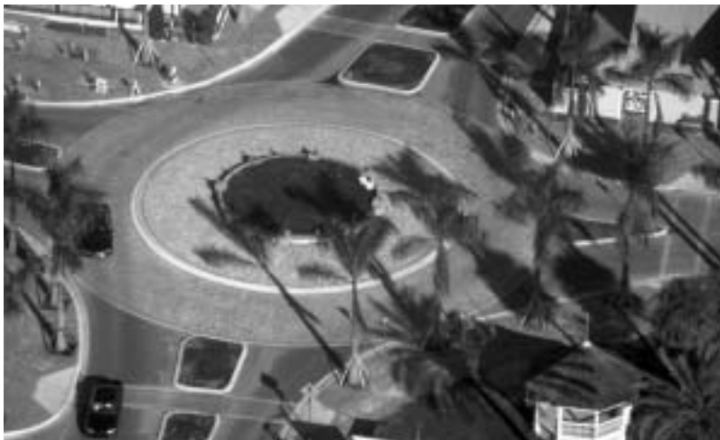
This Fort Pierce, Florida, roundabout is being constructed to reduce speeding, improve safety, and enhance the aesthetics of the community.
